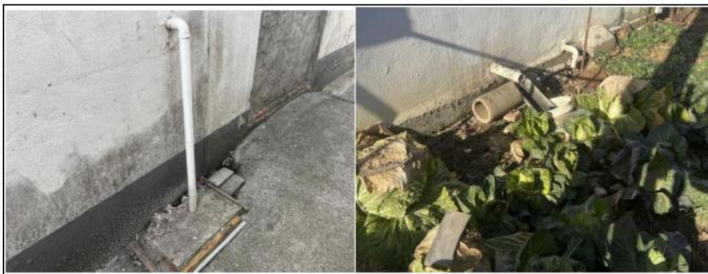
图2.7-4 污水下渗、污水散排现状
