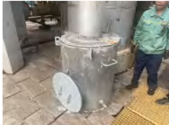
满流槽加盖封闭
