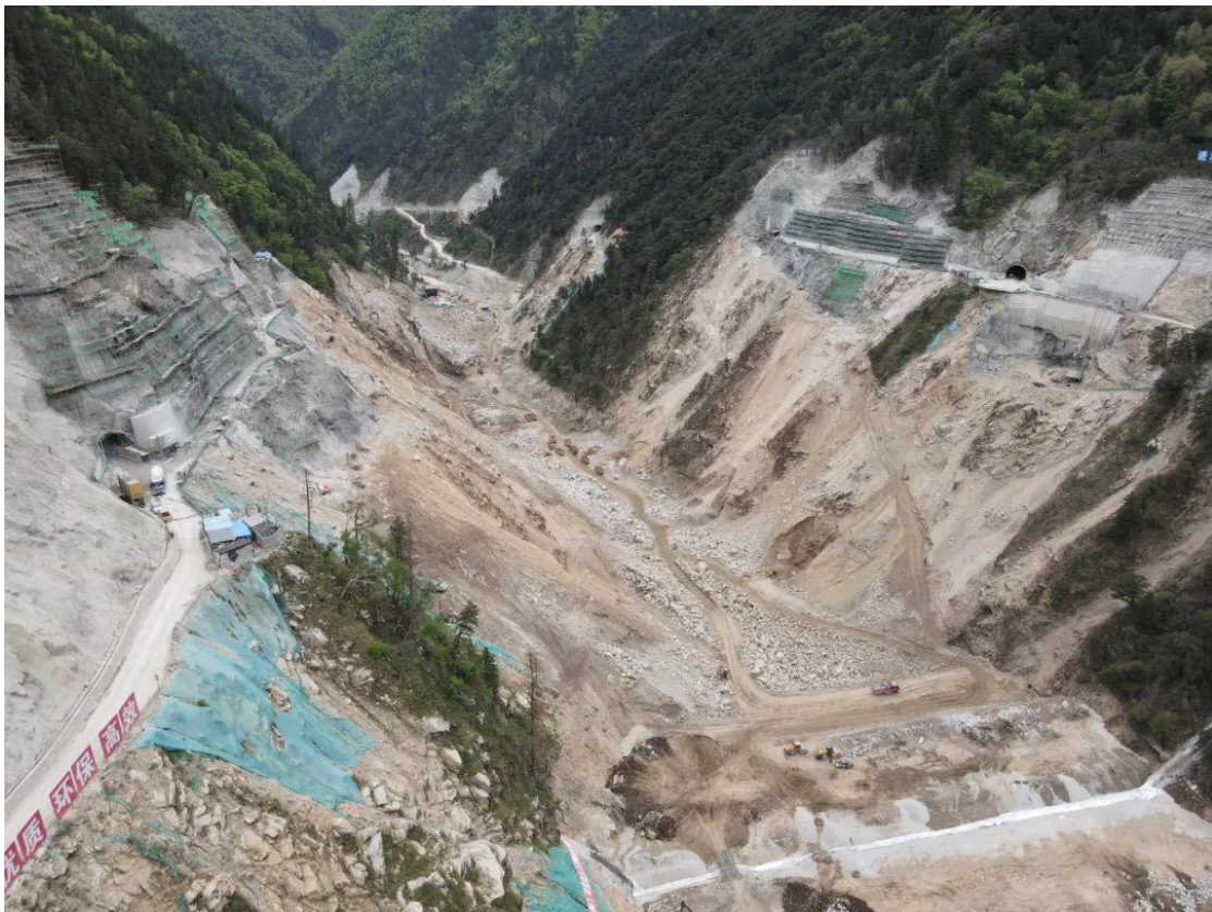
The construction site of the Bara power station
