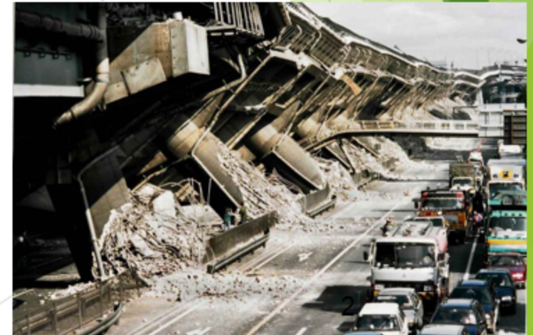
Collapsed viaducts of expressway
