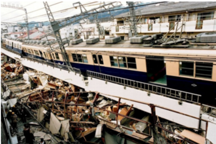
Damaged railway track
