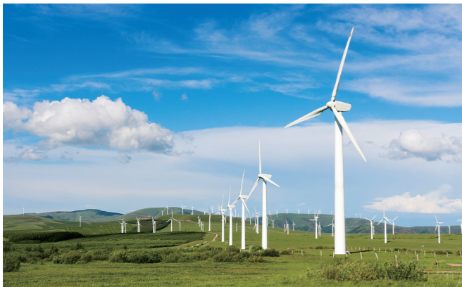
风力发电巡检
