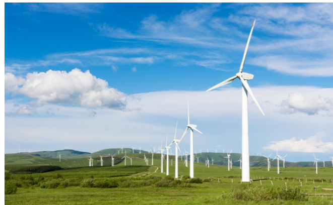
风力发电巡检 Wind blade inspection
