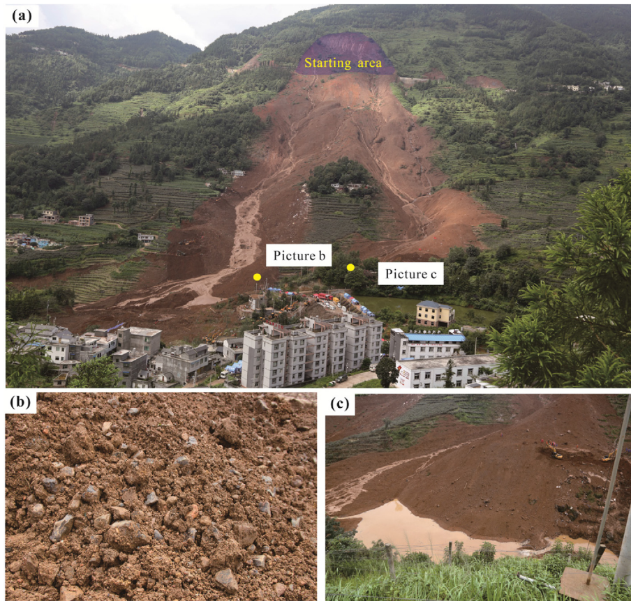
Fig. 10. Situation of the Shuicheng landslide: (a) Full view of the Shuicheng landslide, (b) Image of solid materials mainly composed of basalt debris of 0.1–0.3 m in diameter, and (c) Image of liquid materials mainly composed of slurry mixed with fine grain soil and ground runoff.
