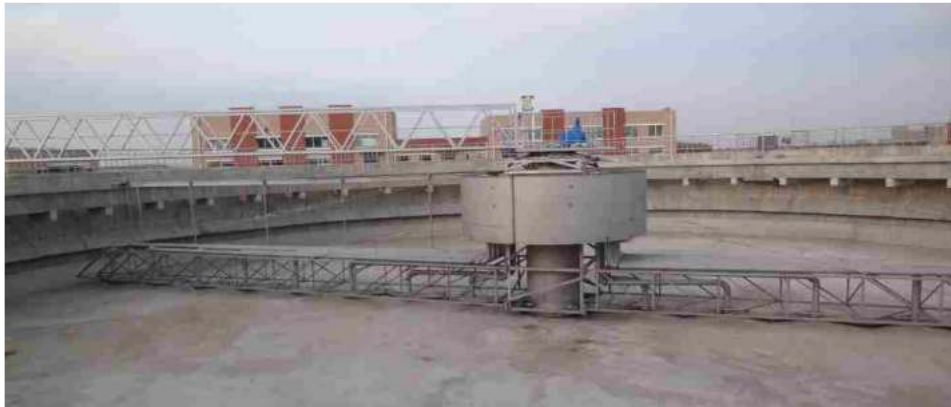
垂架式中心传动吸泥机结构示意图 Hang down posture center sucking machine structure transmission schemes
